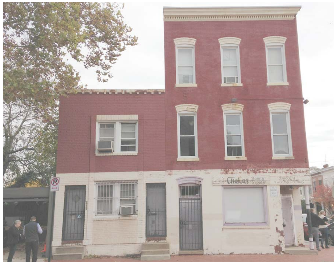
VIEW AT FRONT FACADE
