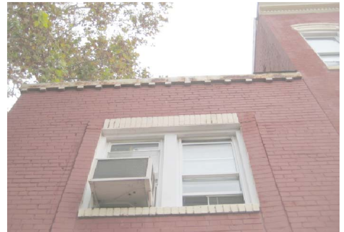
ROOF COPING - EXISTING CONDITION
