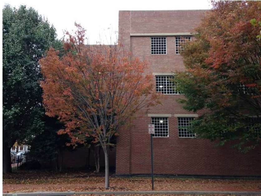
1. 2021 4TH STREET, VIEW WEST
