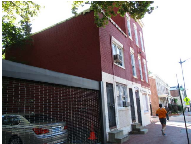
3. 2021 4TH STREET, VIEW SOUTHEAST
