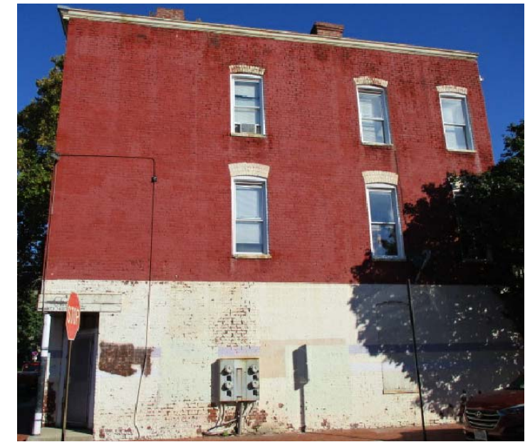
EXISTING BUILDING-SIDE (SOUTH)
